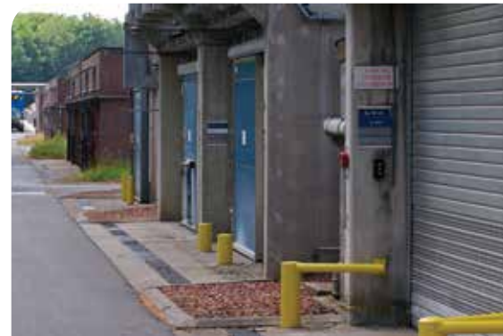
Organic peroxide storage rooms
